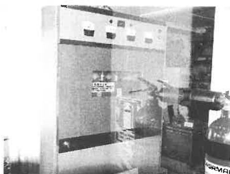
The 1962 vintage Toshiba 1 KW AM transmitter is ex 2YG Gisborne and has had nearly 100,000 hours of service. It uses type 4/400 valves in the modulator and final amplifier.
