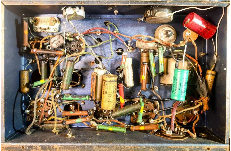
The author's Stella 5A under chassis before repairs
